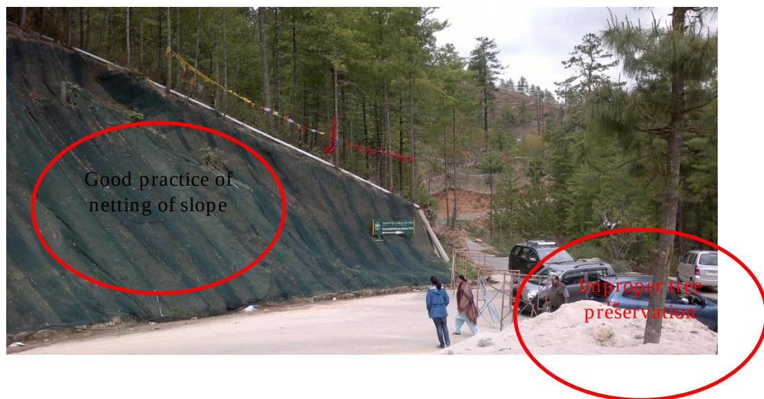
Figure 5: Good practice of netting and anchoring in one of the big construction project
