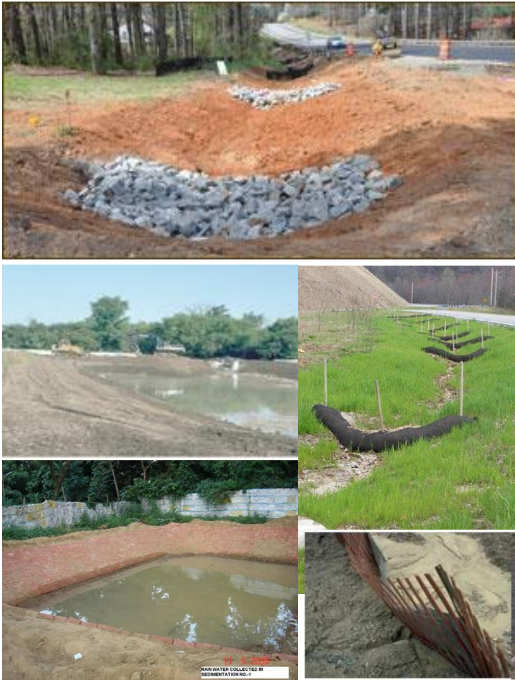
Figure 6 : Some of the soil erosion and sedimentation control strategies
