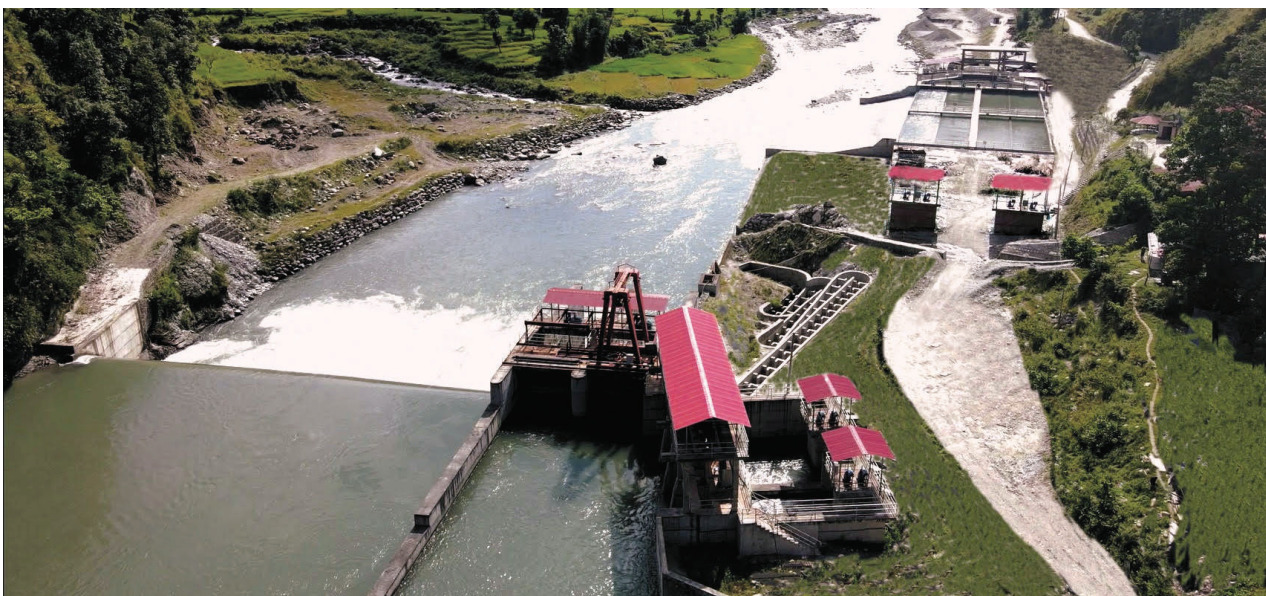
A hydropower project in Okhadhunga district.
