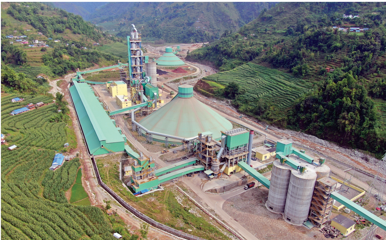
A cement factory in Dhading district.
