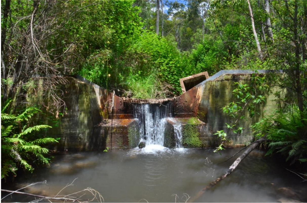
**Figure 4.1** Lees Creek weir is a potential barrier to passage for some aquatic species, reducing connectivity. However, the weir can also form a barrier to pest species invading the upstream river section. Photo: M. Jekabsons, ACT Government.
