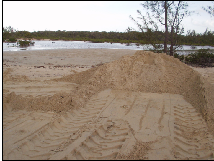
Figure 5: Grading of Land within a Wetland System
