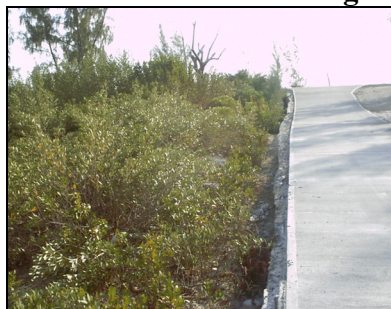
Photo 1: Roadway cutting through the wetlands
