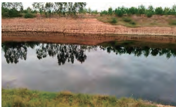
Leachate Management in Dangkor Landfill site
