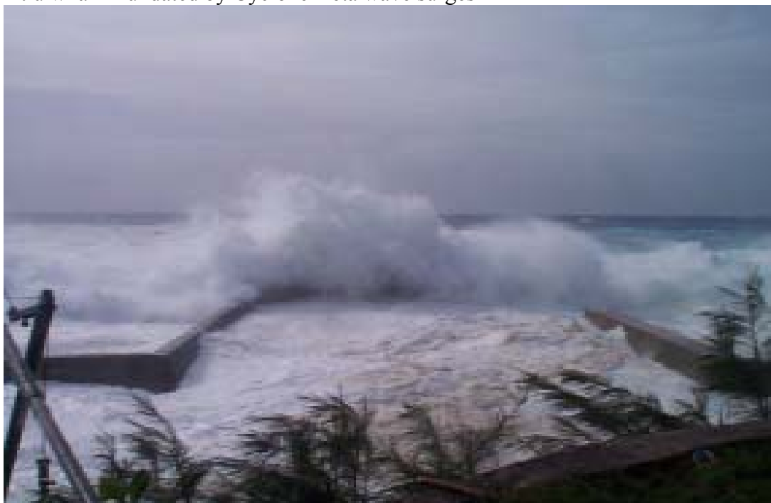
Atiu wharf inundated by Cyclone Heta wave surges
