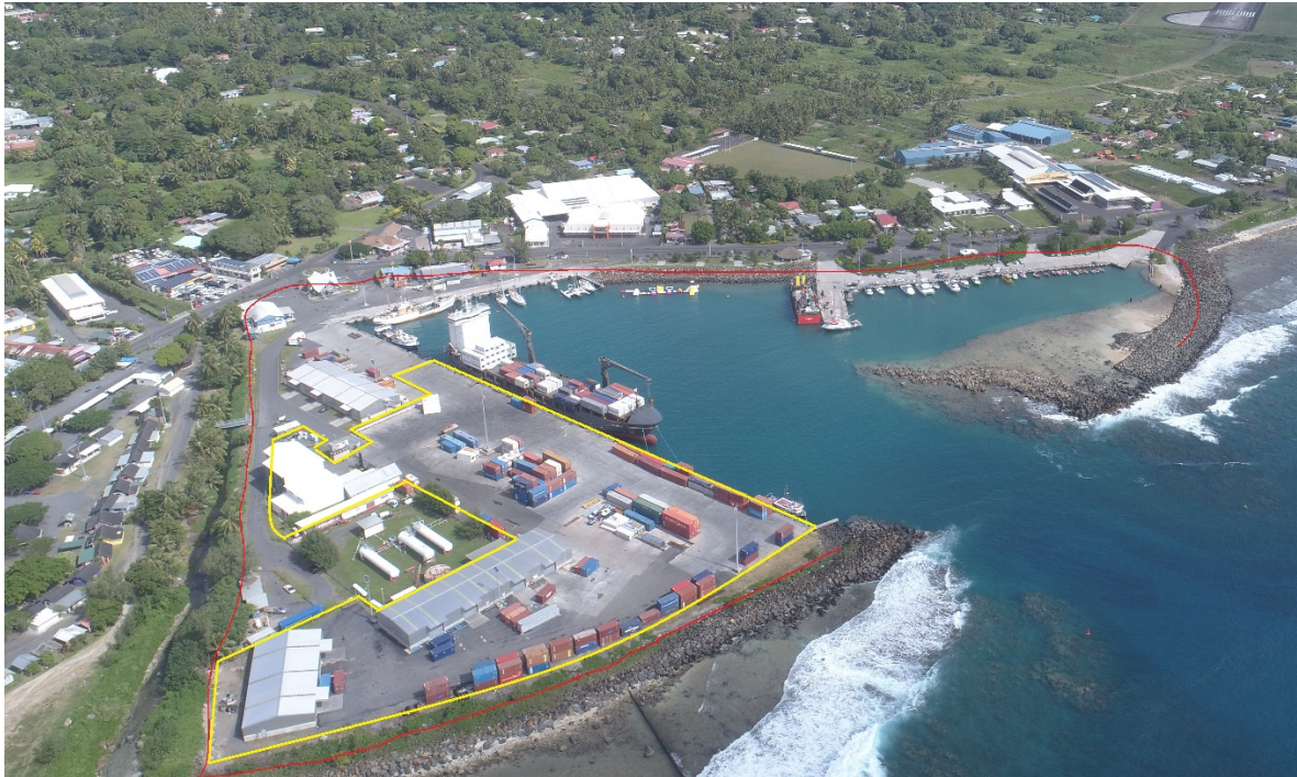
Figure 1: Aerial view of Avatiu Harbour and Port. Image supplied by Cook Islands Ports Authority
