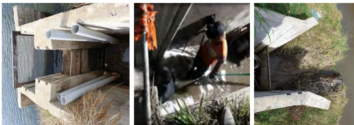
Figure 10. Pictures of the inner, middle and outer sections of a concrete sluice gate at KPFL farm.
