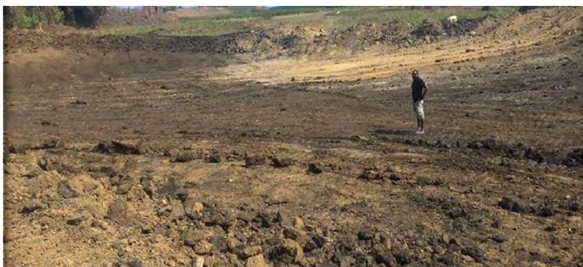
Figure 8. Construction of pond bottom and dyke supervised by Thushan Gunasena, Director KPFL.
