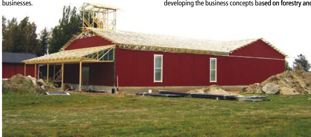
A combined carpenter's studio and shop constructed of Ryhti elements as a turnkey delivery. The size of the building is 600 m 2 . Photo: Tapani Kaipio.
