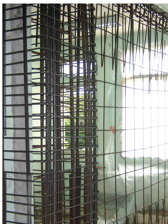
Renforcement parasismique © Vincent Courtray - MEDDE
