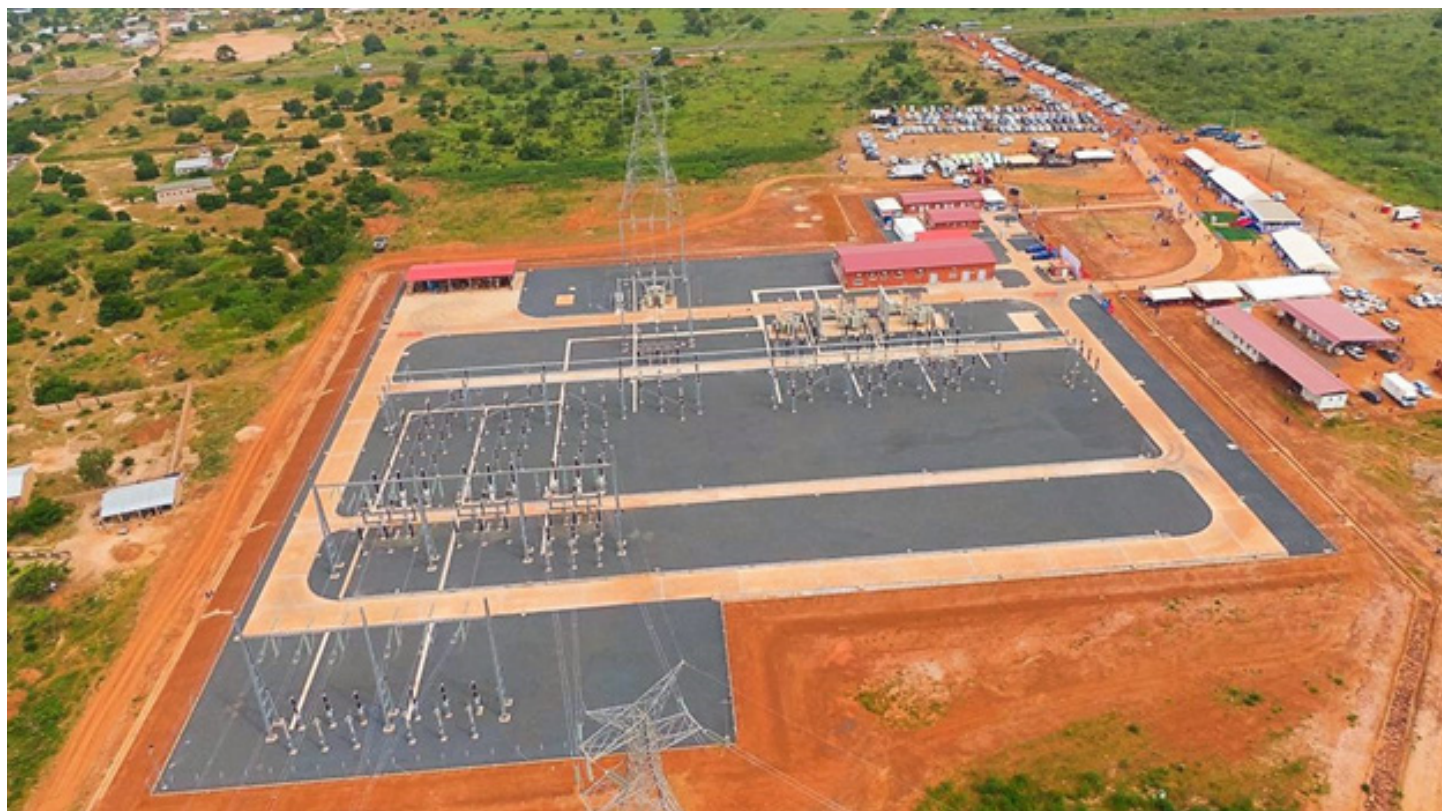
Aerial view of the OMVG substation at Lower River Region (2021)
