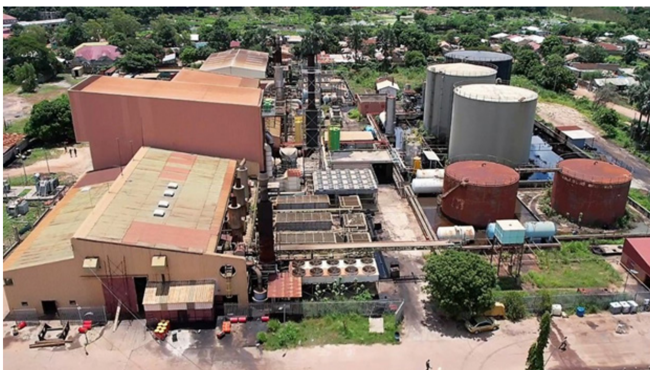
Aerial view of Kotu Power Station, The Gambia's oldest and largest HFO power plant (2022)
