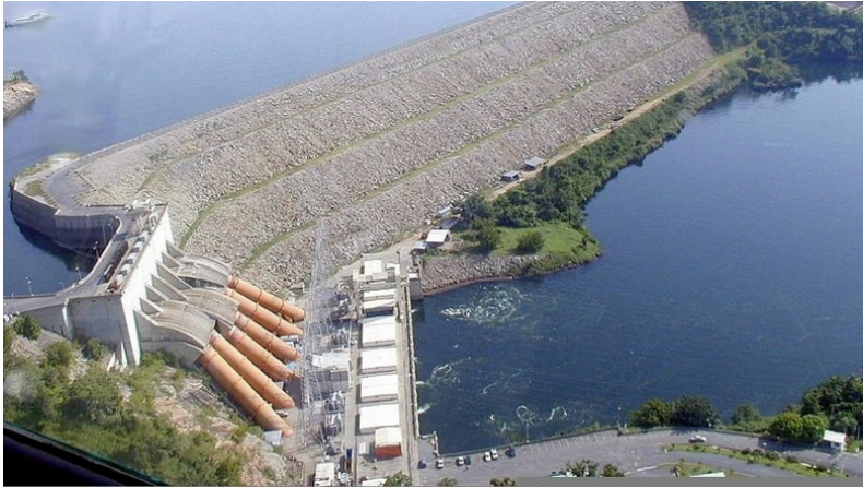
Aerial view of the Akosombo hydro-electric dam
