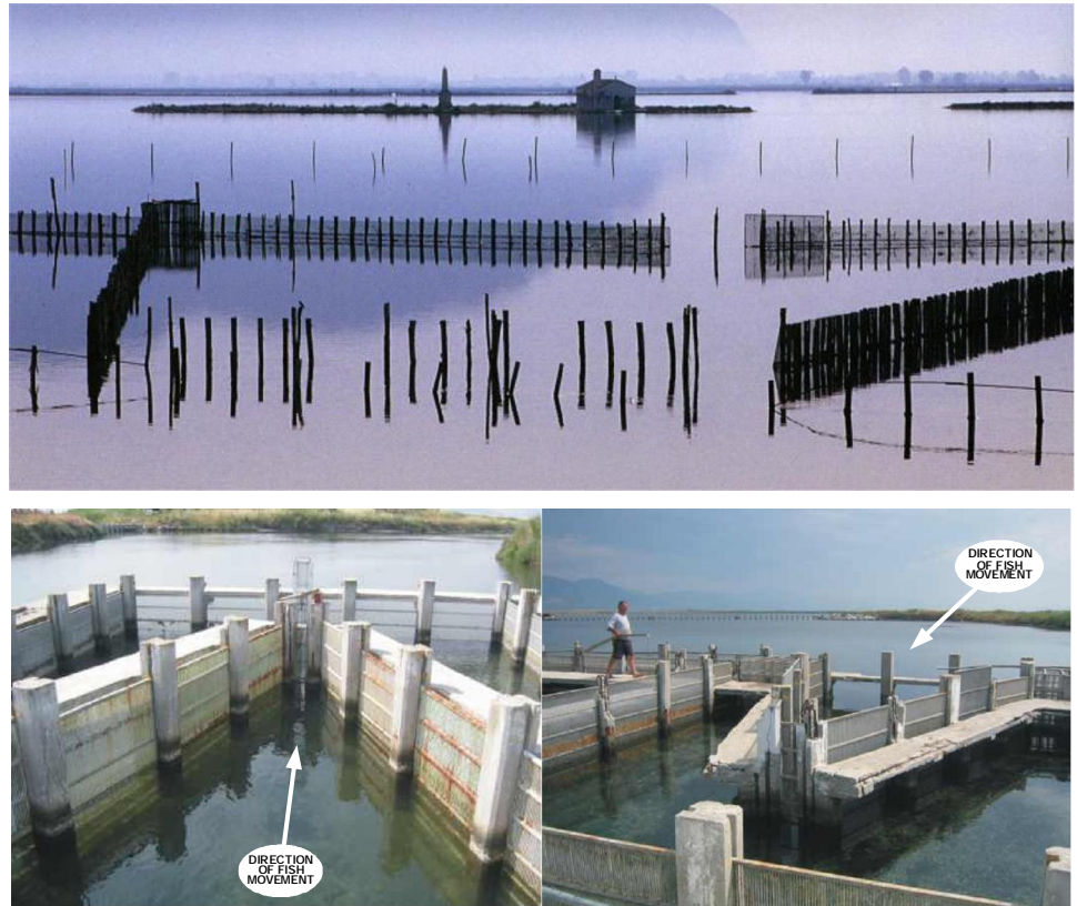
Figure 3. 1 Traditional (above) and modern (below) barrier fish traps installed in Greek lagoons (Source: Koutrakis et al., 2007)
