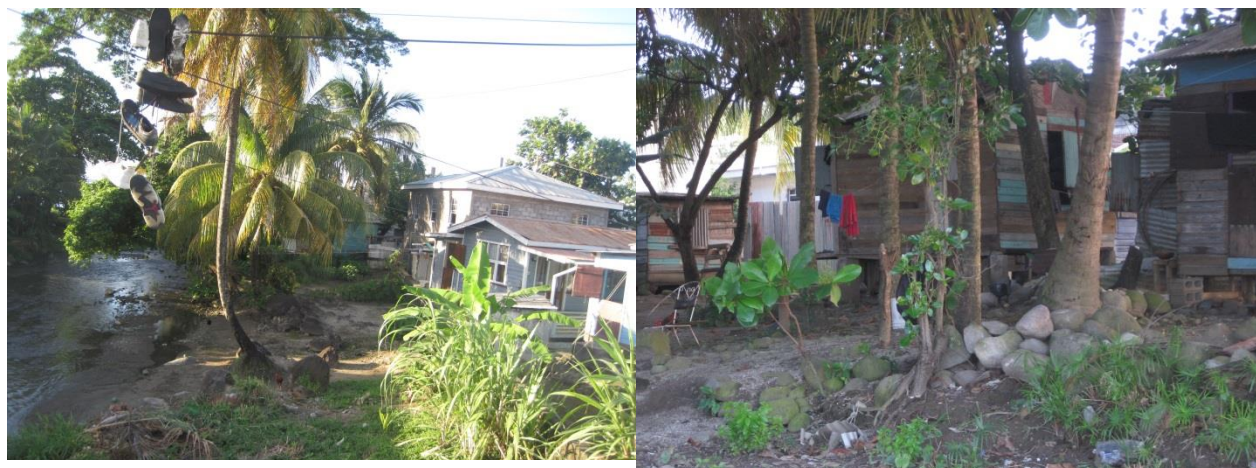
Photo Plate 1.1.7-1: Houses exposed to flood waters along the lower reaches of the Little River, Gouyave, St. John's
