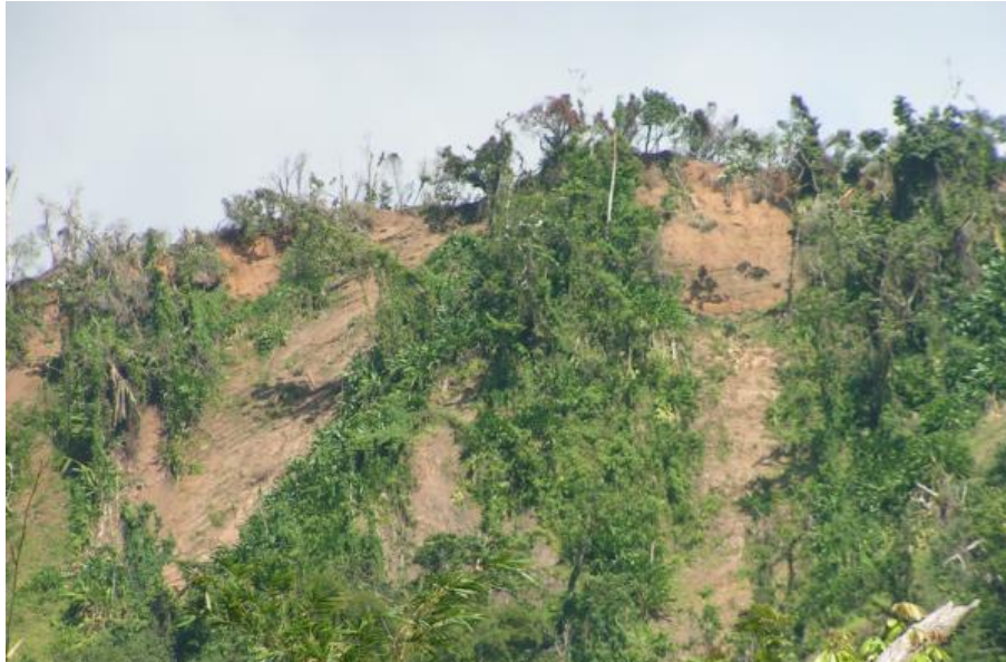
Photo Plate 1.1.2.1-4: Landslide due to Hurricane Ivan in hill slope area
