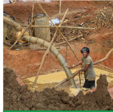
3) The slurry is directed to the marack hole via sloping channels. Marack pump and suction hose operated by marack man
