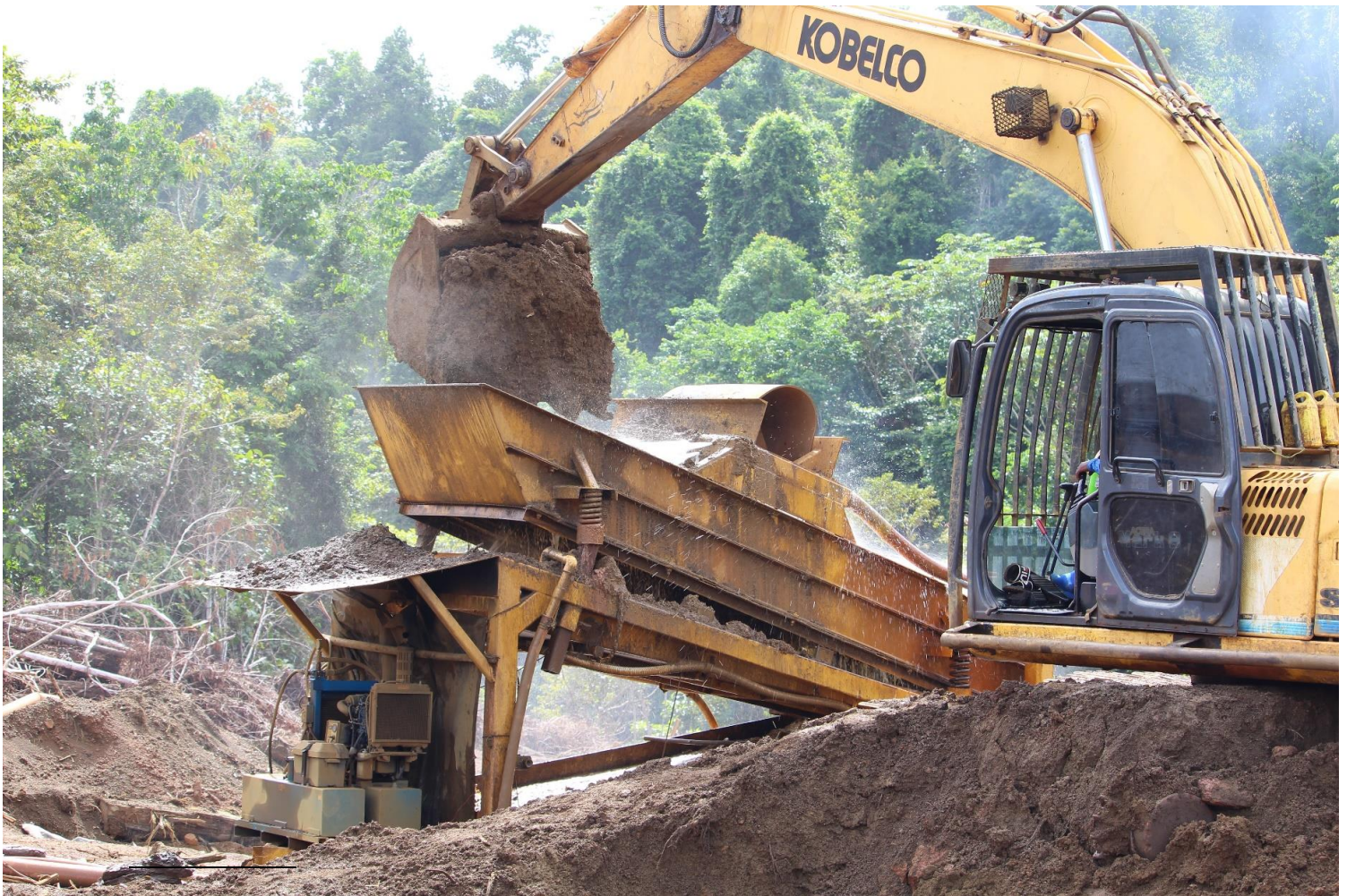
Figure 8: Excavator loading ore onto vibrating screen and built in spurting jets wash materials into a slurry at Puruni (Source: BCRC-Caribbean)
