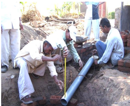
The pipe should have adequate slope
