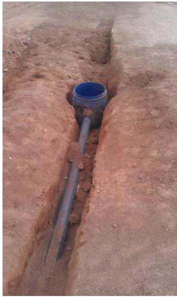
Bucket being as a septic tank, fed into by stolen piping
