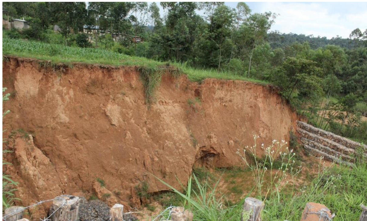
Figure 25: An image of a landslide at Madira village in Lugaga/ Wamuluma Ward.
