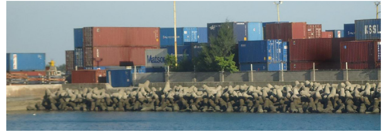
Container Yard, Kiribati Ports Authority
