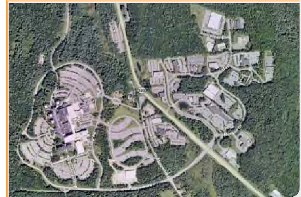
DHMC and Route 120 development 1992 (above) and 2009 (below)
