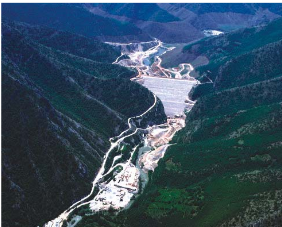
Figure 121. Kozyak Dam (in construction) (Photo: M. Dzingo)
