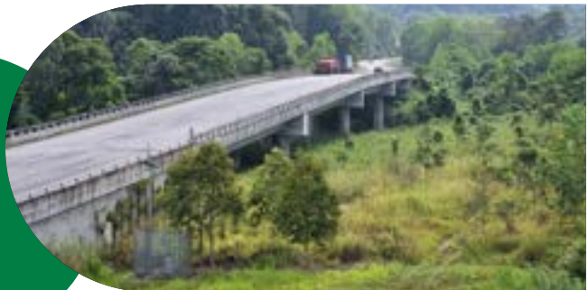
Figure 32: Viaduct in Gerik, Perak (CFS 1 PL 2: Temenggor FR – Royal Belum State Park) completed in 2015 that cost RM25 million
