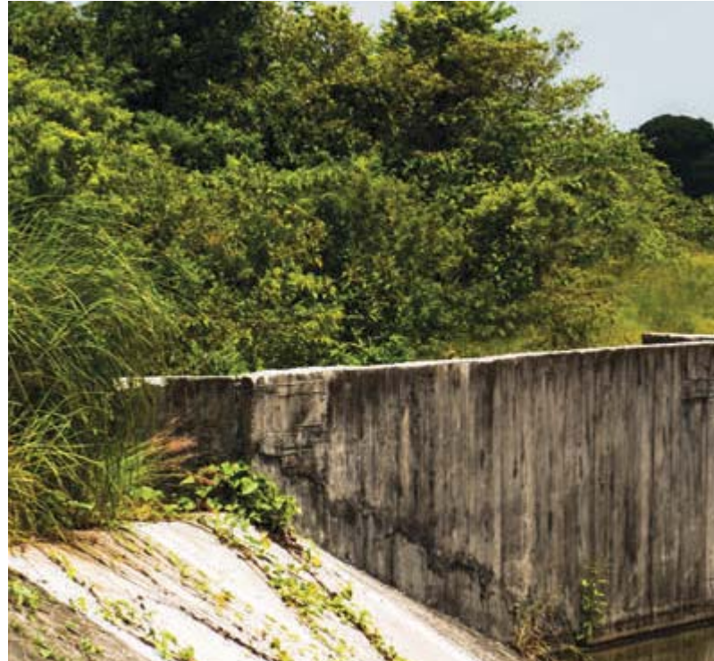
Conveyance channel, La Cangrajera Dam, Veracruz.
