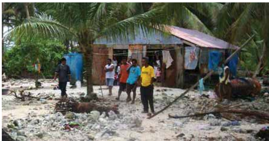
Figure 4: Damage from high sea surge, Lekinioch, Chuuk Source: Pacific Climate Change Science Program partners 2011/
