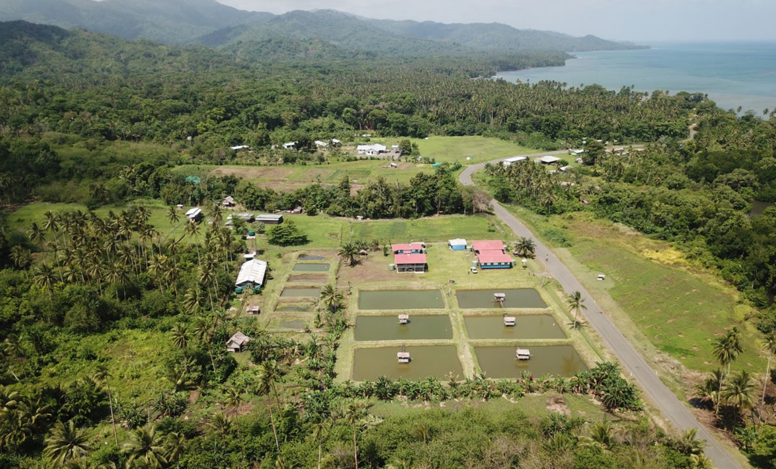
Bubuleta Tilapia Hatchery Facility, Alotau, Milne Bay Province
