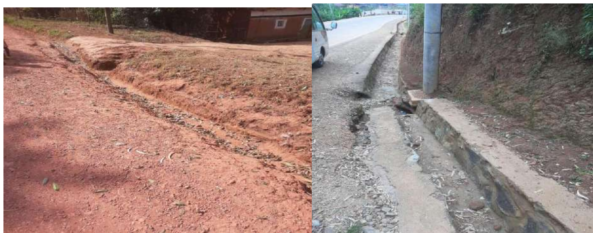
Figure 24. improper road drainage channels in rural area and urban
