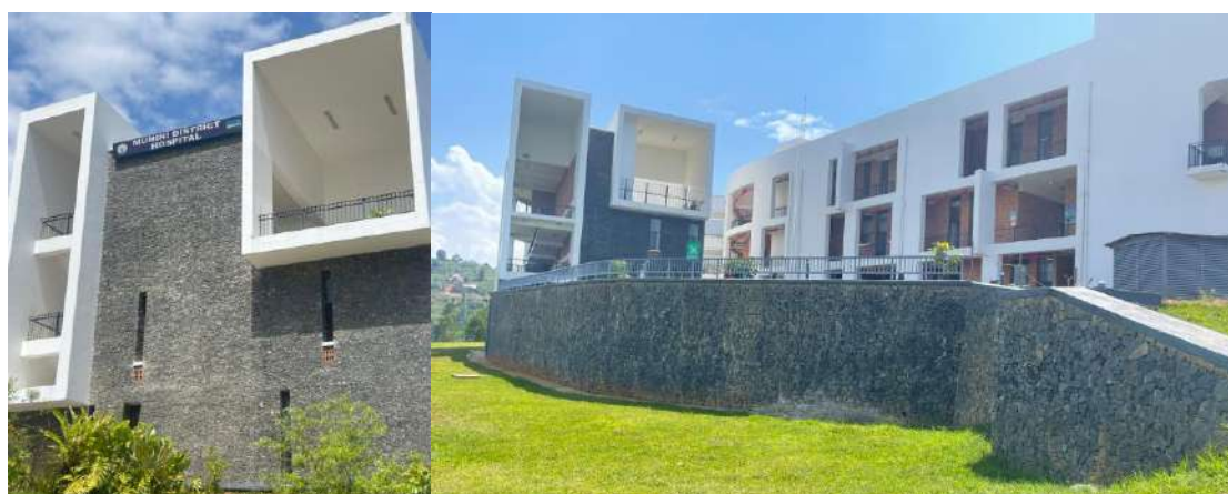
Figure 17: Munini District Hospital
