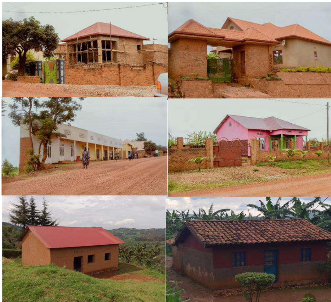
Figure 17: Existing Houses (Source: Photos taken by Author in Ruli sector, 2022)
