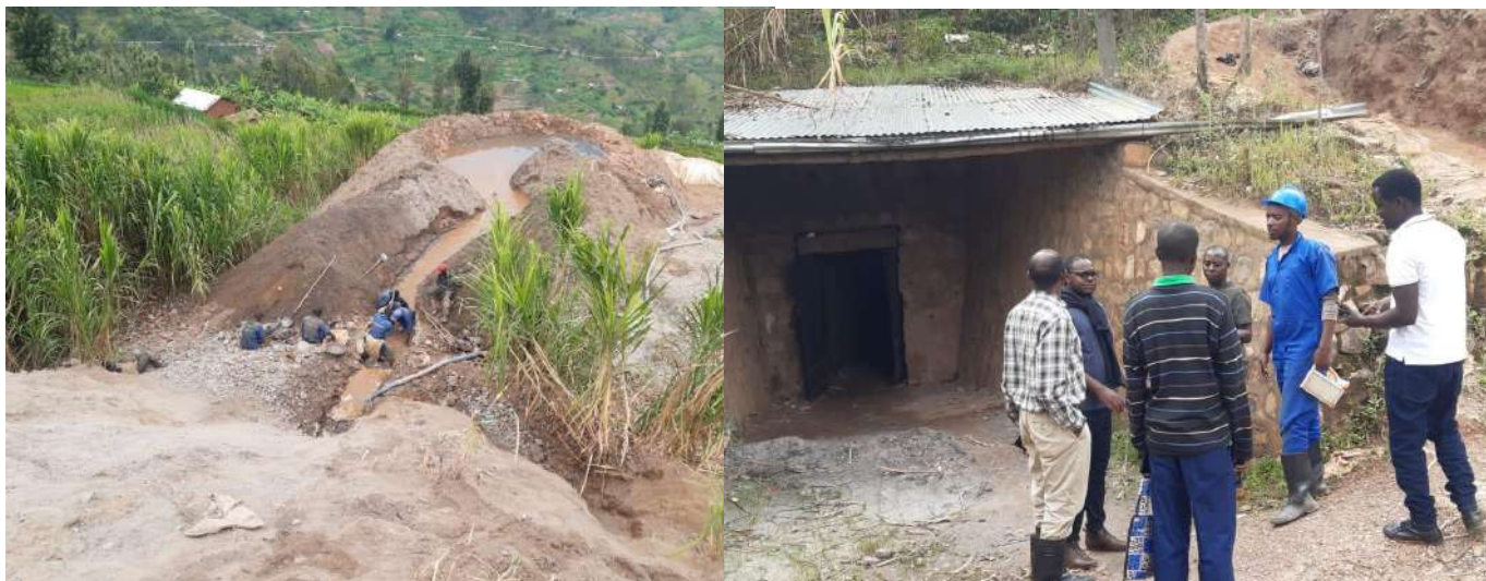
Figure 25: Mining activities Photos (Source: Photos taken by author in Ruli sector, November,2022)
