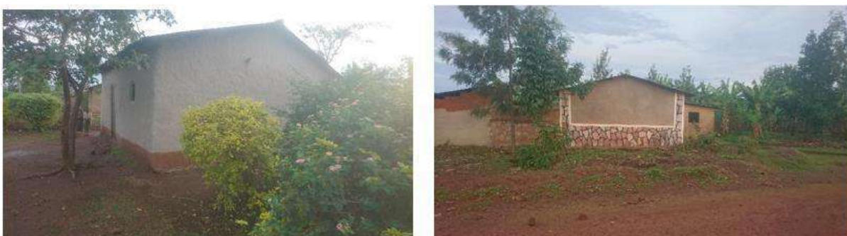
Photo 10: Plastering and Stone Cladding in Ngoma District-Source: Field photos, September 2022
