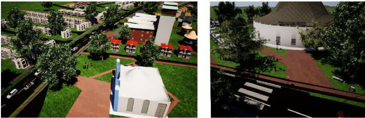
Figure 24: Religious Facilities: Sake Mosque and Cultural Center
