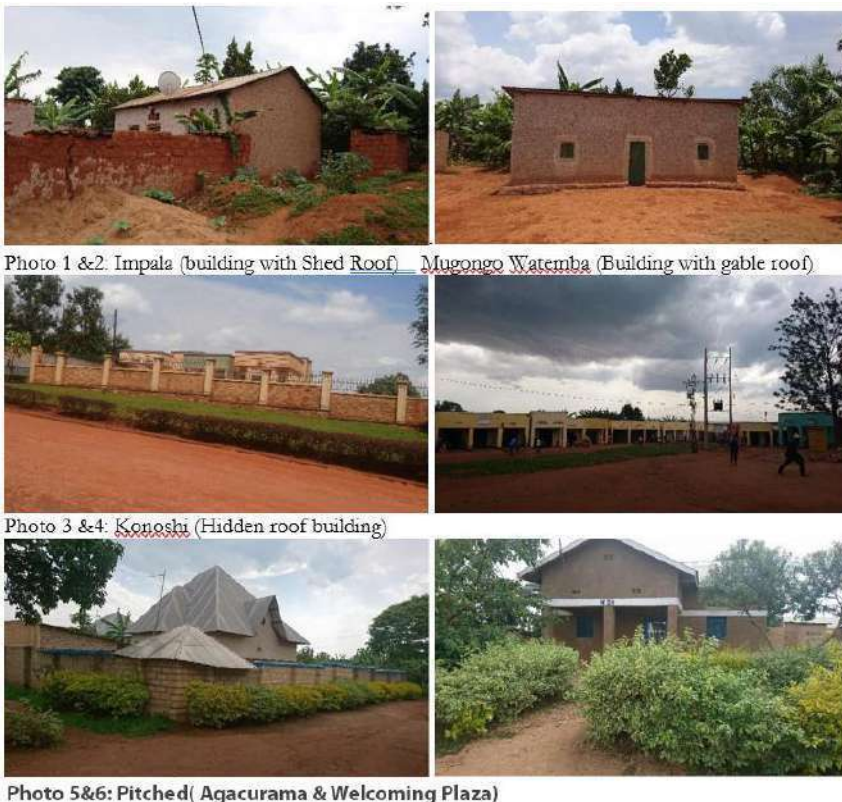
Figure 11: Photos illustrating existing Building in Ngoma District
