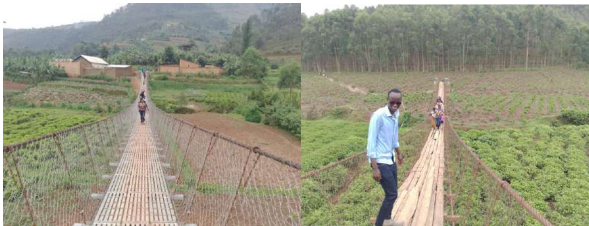
Figure 26. Rulindo District suspended Bridges
