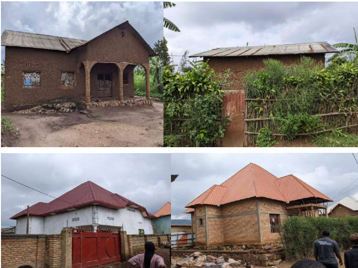
Figure 15. Existing condition of Rulindo houses.
