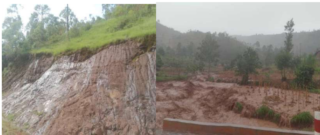
Figure 43. Pictures showing environmental hazards in Rulindo District.
