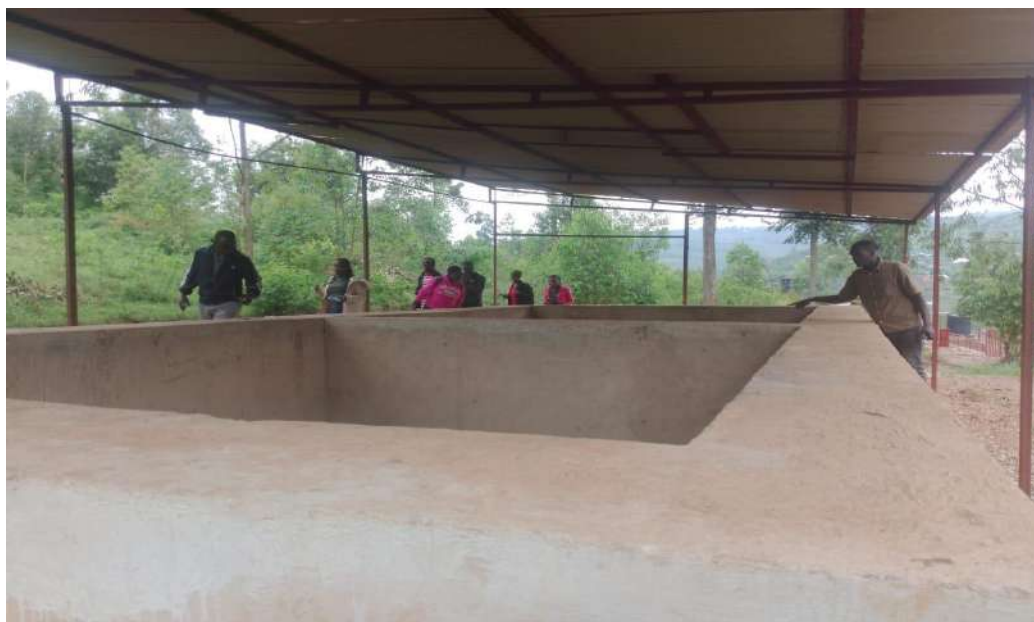
Figure 46. Construction of disposal site of Rusine Market in Masoro Sector
