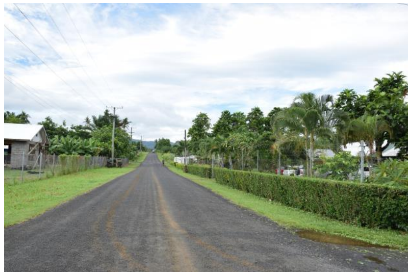
Plate 4: New Subdivisions – sealed roads
