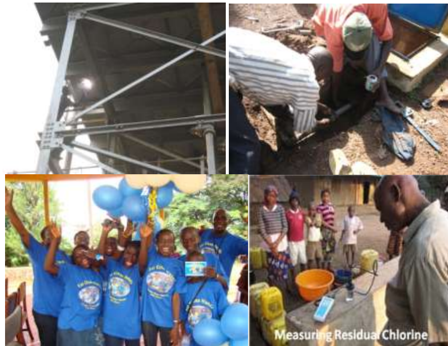
Installations, Repairs, Testing and Training Activities
