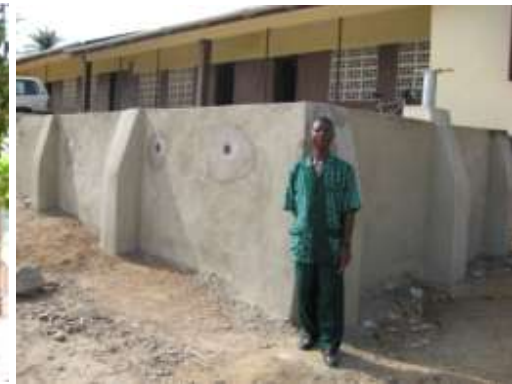
School Rainwater Harvesting Tank
