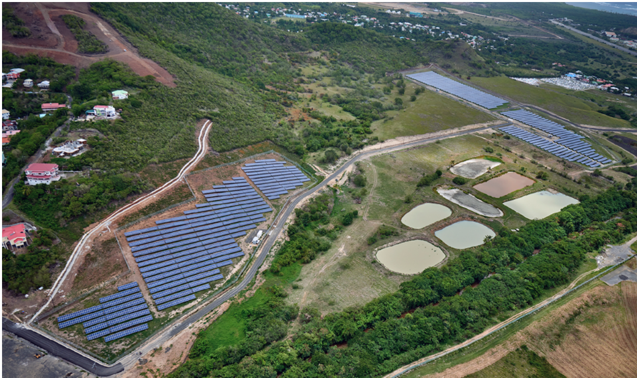
Photo: St. Lucia Electricity Services, Limited
