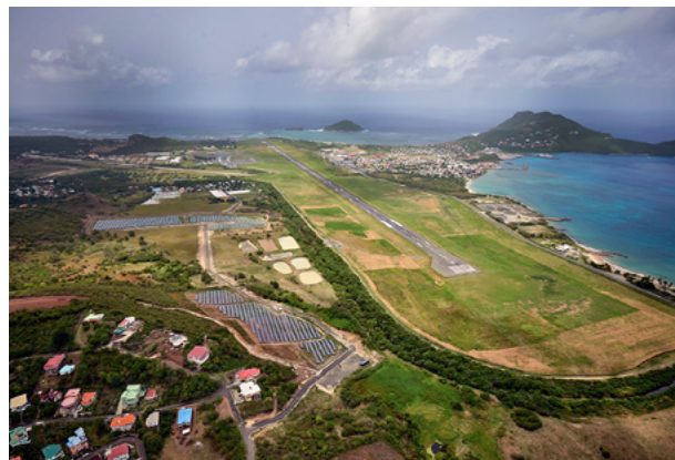
Photo: Saint Lucia Electricity Services, Limited
