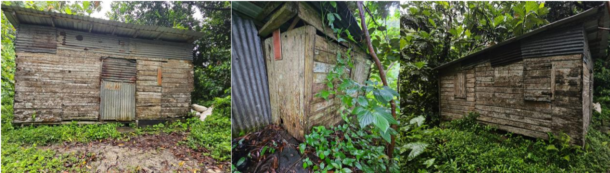
Figure D-5: Material Storage Shed Owner: SLC-01
