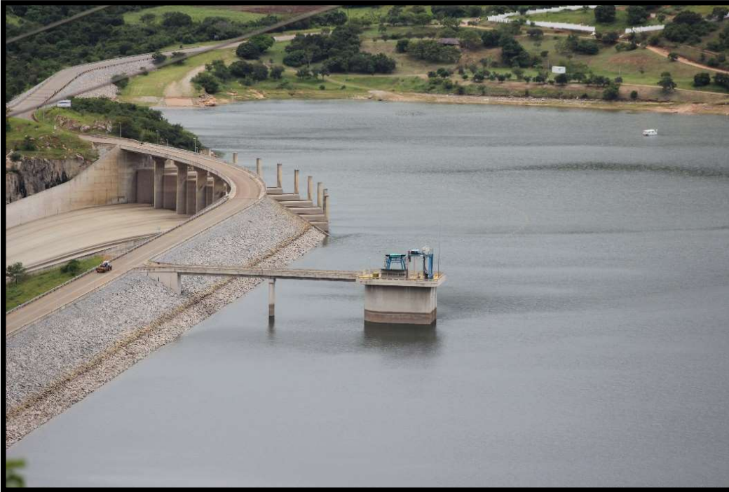
FIGURE 5 AERIAL VIEW OF THE MAGUGA DAM ON THE KOMATI RIVER
