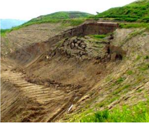
Proper cutting of earth materials during construction
