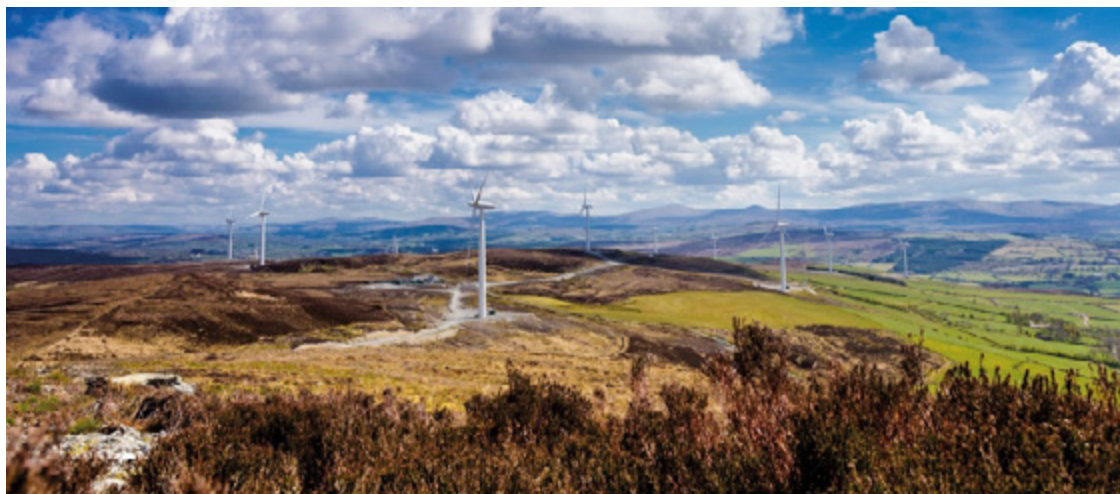
Image 4-2: Slieve Kirk Wind Farm (SSE Renewables)
