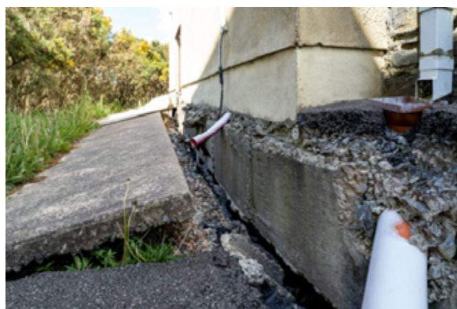
Image 5-6: Impact of subsidence on a residential property (Claim Management Group)
