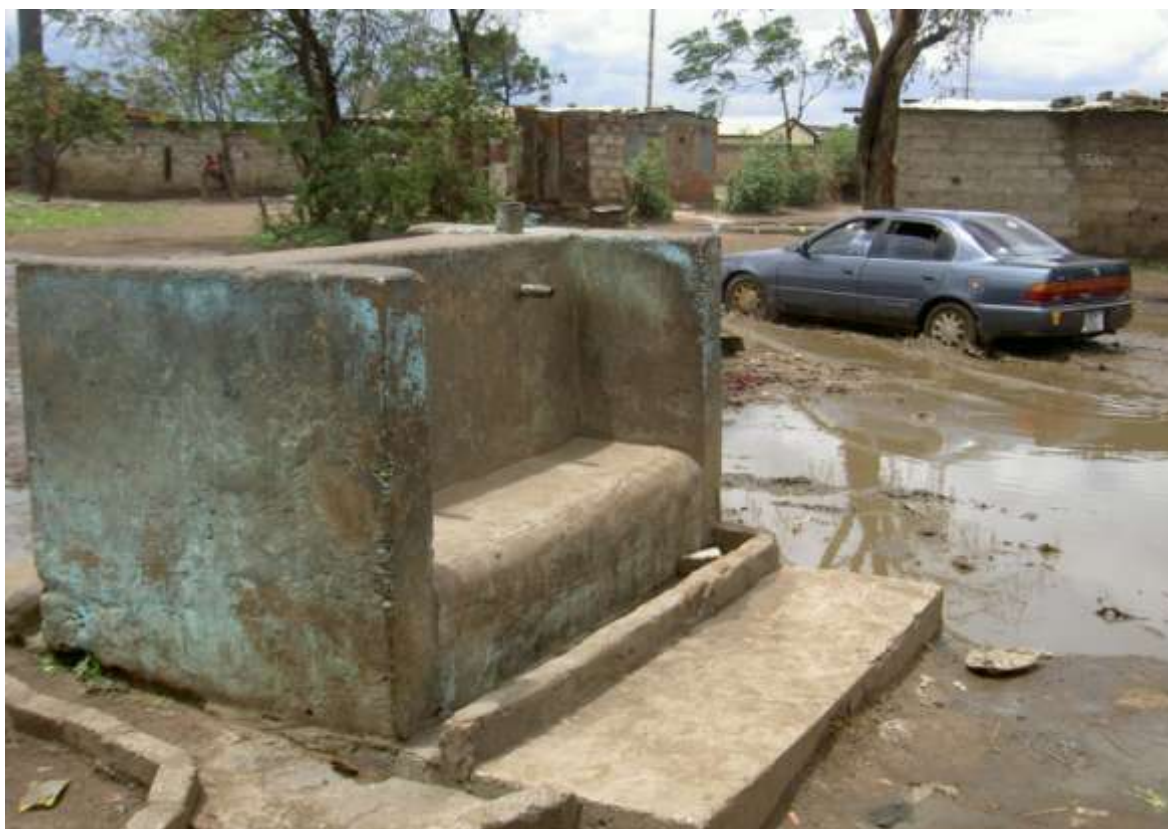
Typical drainage challenge aimed to be addressed in NUWSSP
