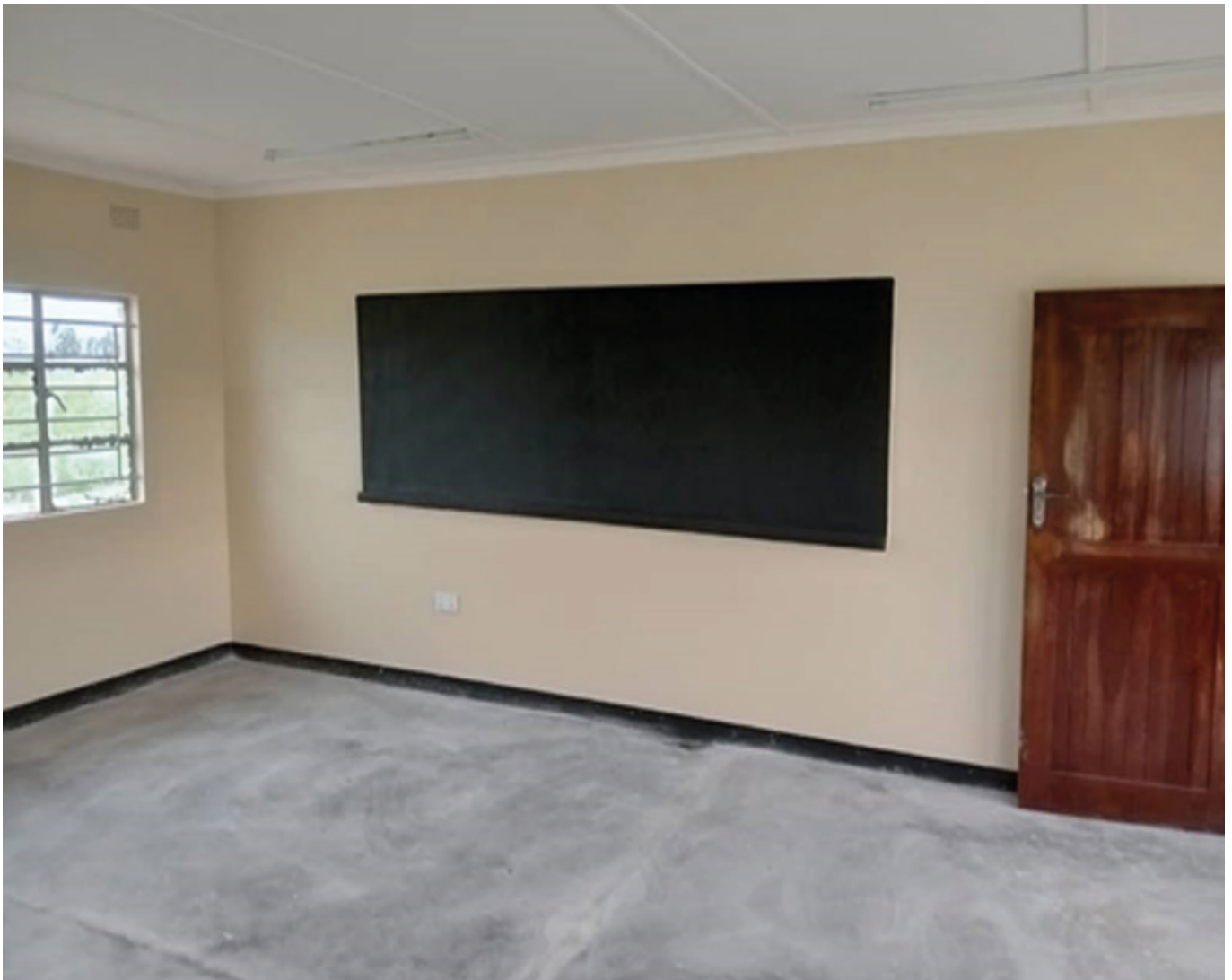
Constructed 1x3 Classroom Block at Natuseko School under CDF
