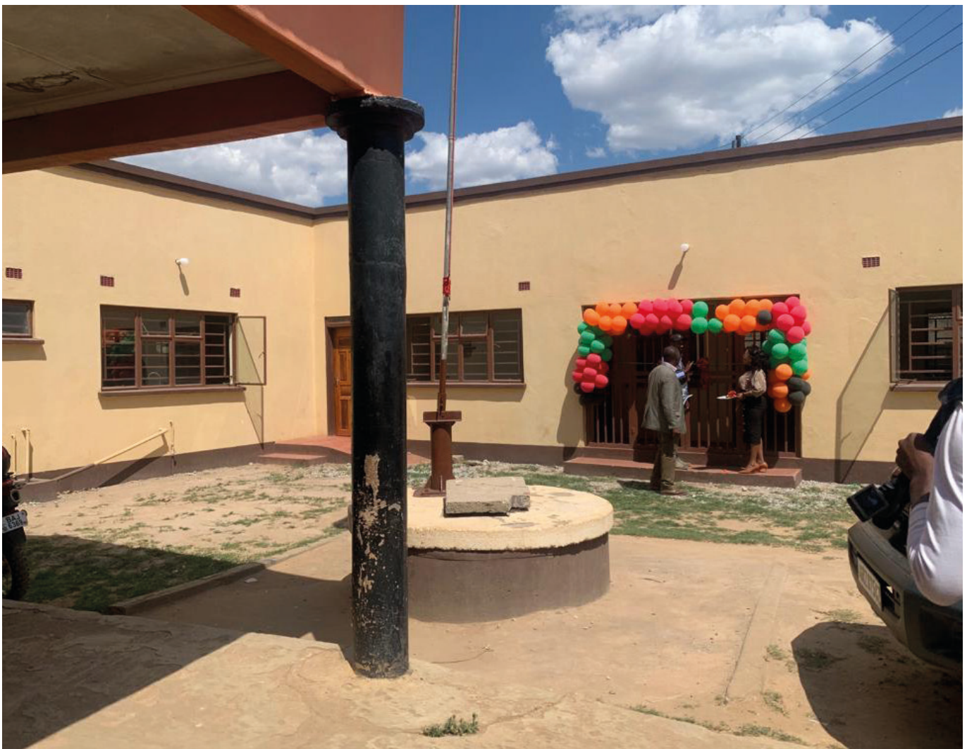
Constructed maternity annex at Nakoli clinic under CDF
