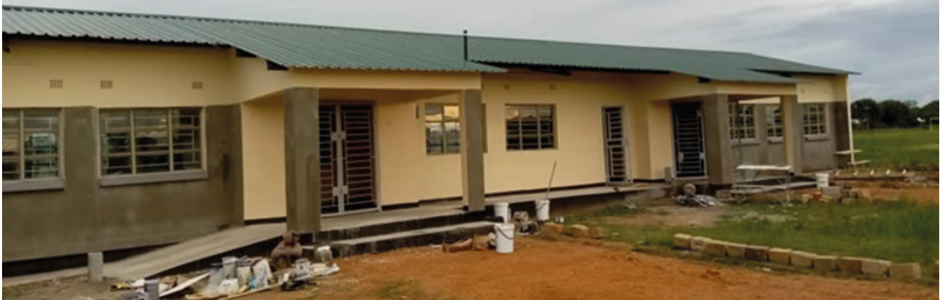
Constructed 1x3 Classroom Block at Natuseko School under CDF
