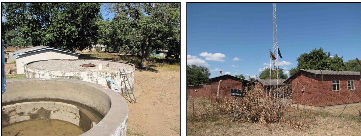
Figure 53: ZINWA and Police infrastructure at Nyamepi
