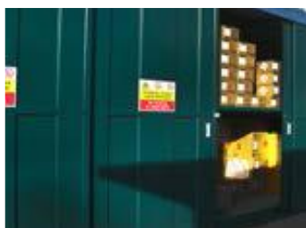
Storage of chemicals in different safety compartments
