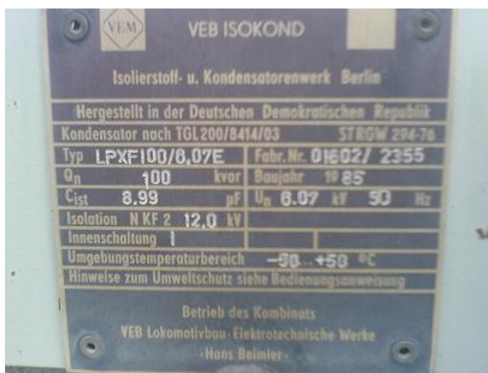
Image 4: Manufacturer sign of a German PCB capacitor (city substation) operated in Bulgaria
