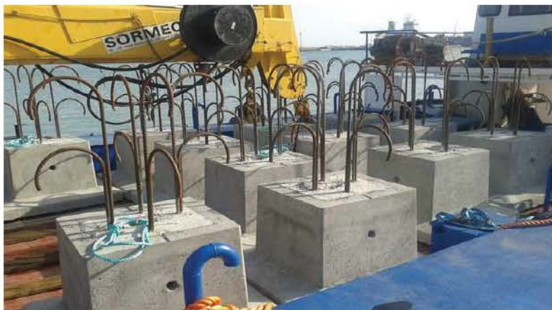
Figure 6: Concrete blocks used for preventing fishing gear
