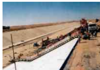
Lining of canal in Toshka project
