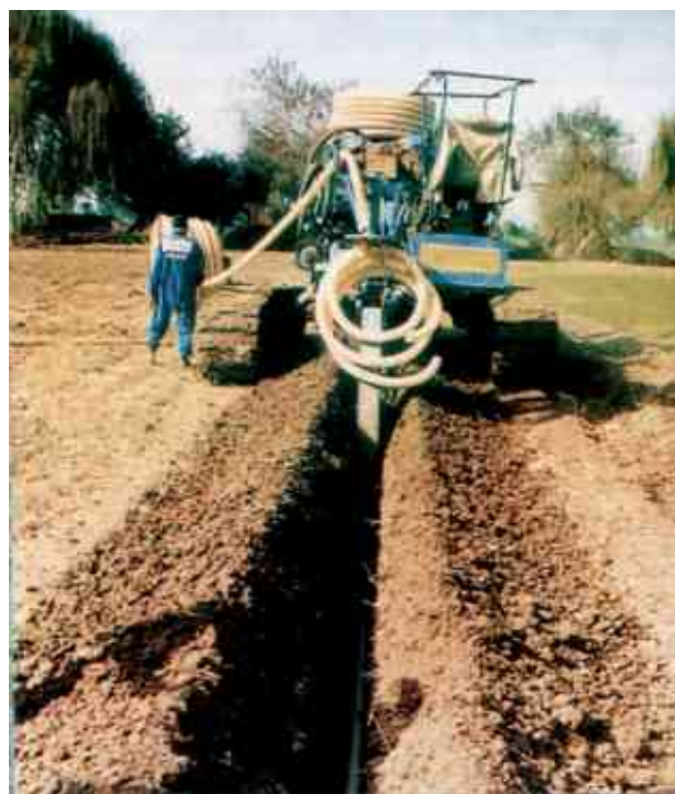
Installing Subsurface Drainage
