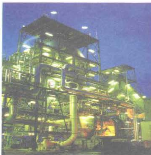
Pusat Pengurusan Bersepadu Buangan Terjadual Integrated Scheduled Waste Management Centre.
