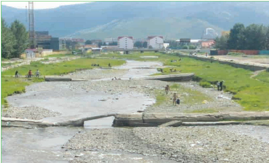
Figure 71. Flood protection channel in the Selbe River
