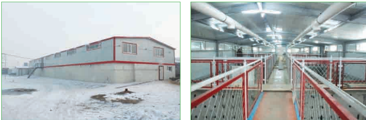
Figure 67. Newly established wastewater pre-treatment plant of Future Holding LLC
