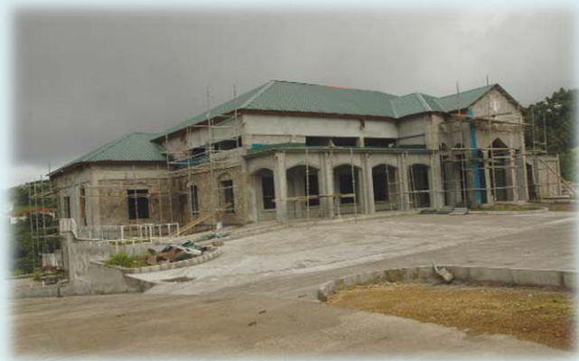
Bank of Montserrat during Construction
