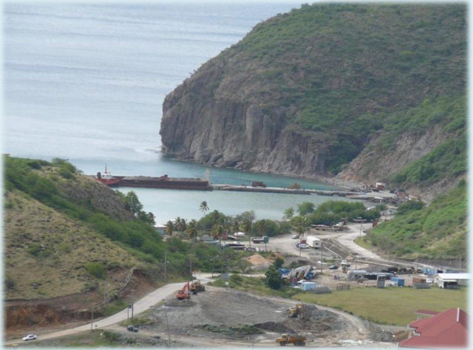
Construction at Little Bay
