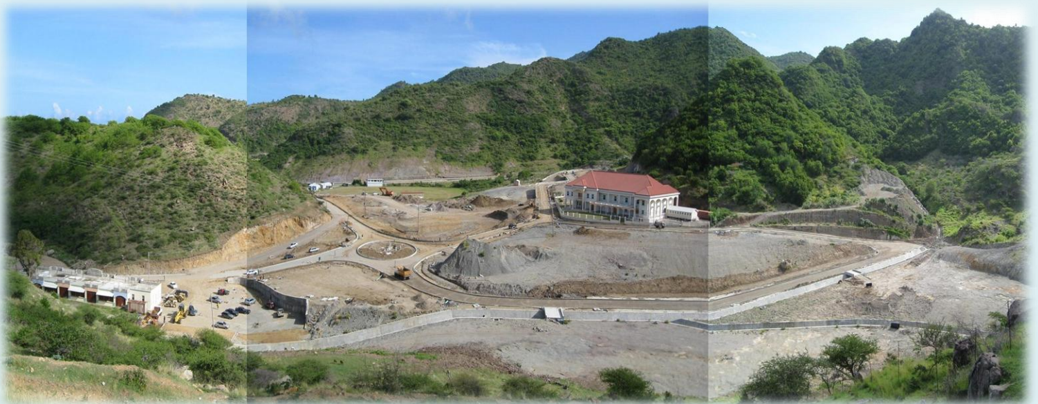
Little Bay Town Centre under construction
