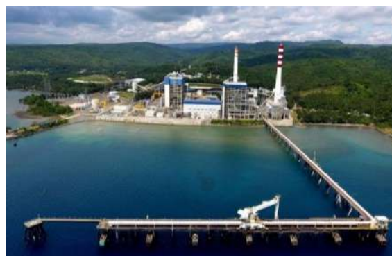
The 500-MW supercritical coal-fired power plant of San Buenaventura Power Ltd. Co. in Mauban, Quezon (source: tribune.net.ph)
