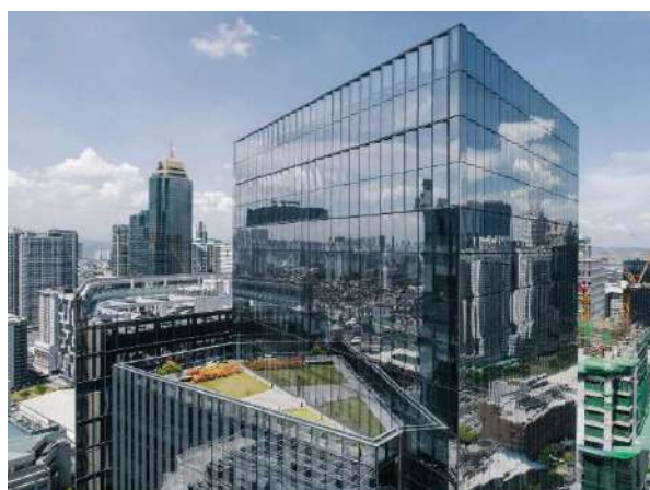
ARTHALAND Century Pacific Tower (ACPT), a mixed-used commercial building located in Taguig business district, is the first in the world to receive EDGE Zero Carbon Certification. The tower has offset 100 percent of its operational emissions and with projected energy savings of 45.0 percent (Source: EDGE Buildings Facebook page)
