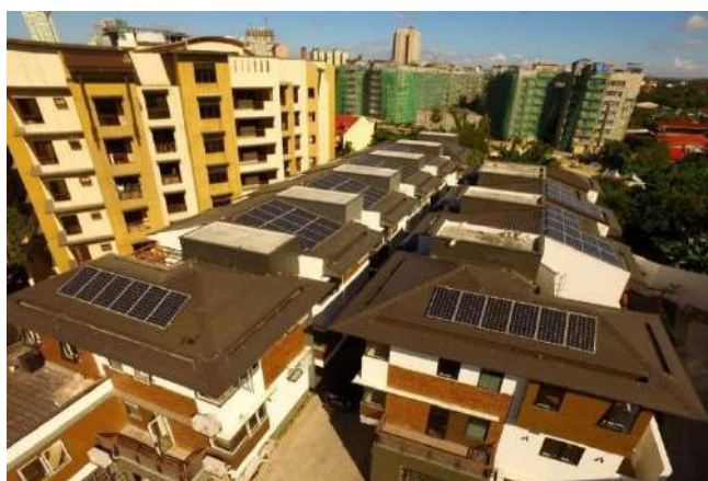
TOWNHOUSES WITH SOLAR ROOFTOPS. Solar installed rooftops are gaining popularity among households that seek to minimize their electricity bills (Source: Solaric Corporation Philippines)
