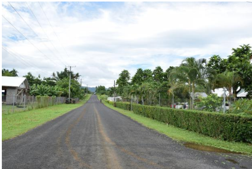
Plate 4: New Subdivisions – sealed roads
