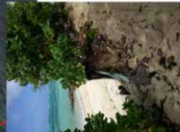
Detail of revetment in the active beach profile that induces erosion.
