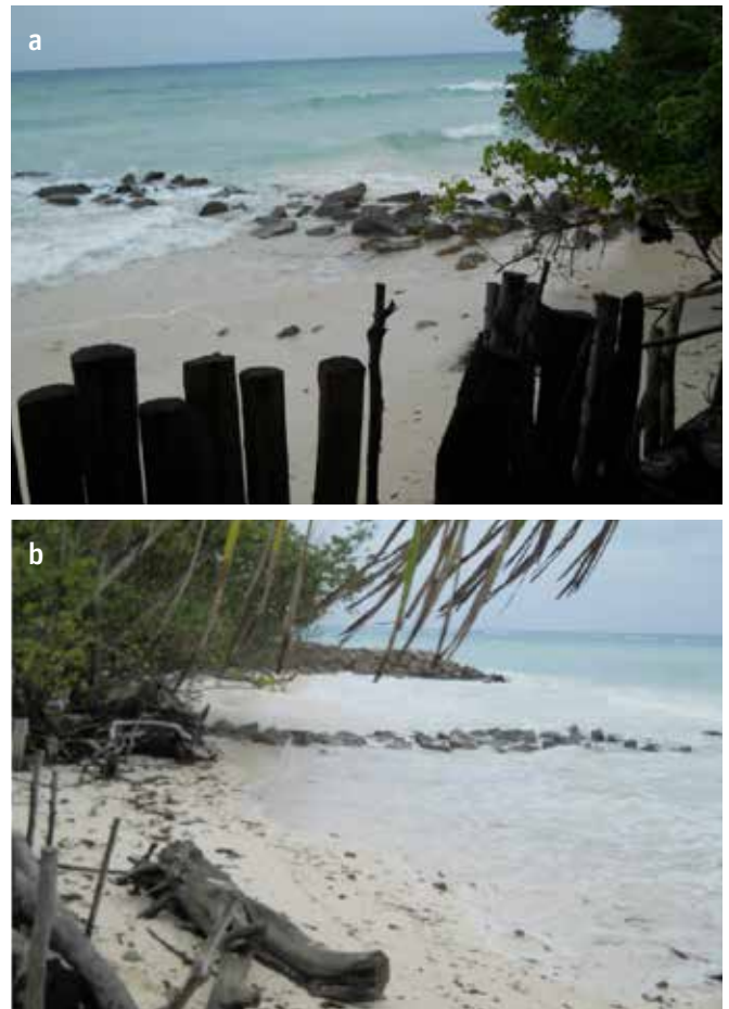
Photo 3.1: Examples of Extreme Erosion in Praslin.
