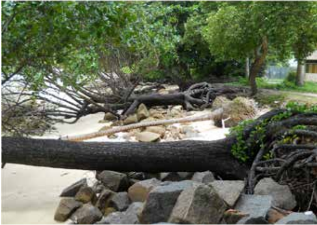
Photo 3.2: Example of Beach Erosion and Rock Armouring Collapsing in the South of Anse Royale.
