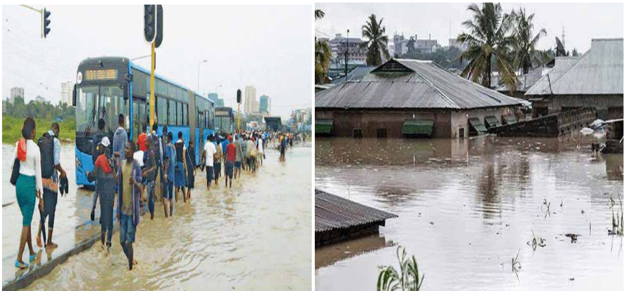
Photo 6: Effects of flooding on road infrastructures, public transport and housing in Dar es Salaam city
